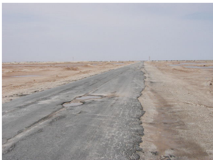
Picture 1.3: Bypass road in Nouakchott.
